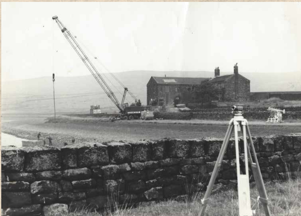
Morley Corporation Withens Reservoir, a large machine on site with a 120 ft. arm reaching down into the core centre of the dam
